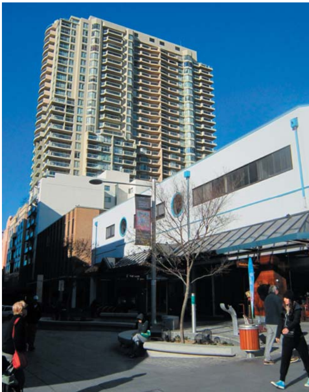
Figure 15 – Upper levels of the Sebel (northern elevation)
