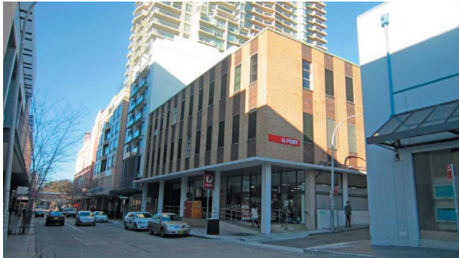
Figure 4 – Victor Street elevation of the existing building
